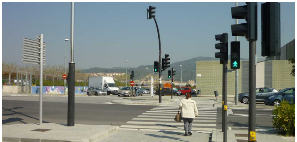
Image 10 Pedestrian crossings of the BV-2002 through road in Sant Vicenç dels Horts have been adapted
