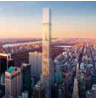
432 PARK AVENUE Institution Responsible: CIM Group / Macklowe Properties Time Frame: 2009 - 2015 Design/Engineering: Rafael Viñoly and SLCE Architects, LLP and WSP Group Size: 426.1 m high
