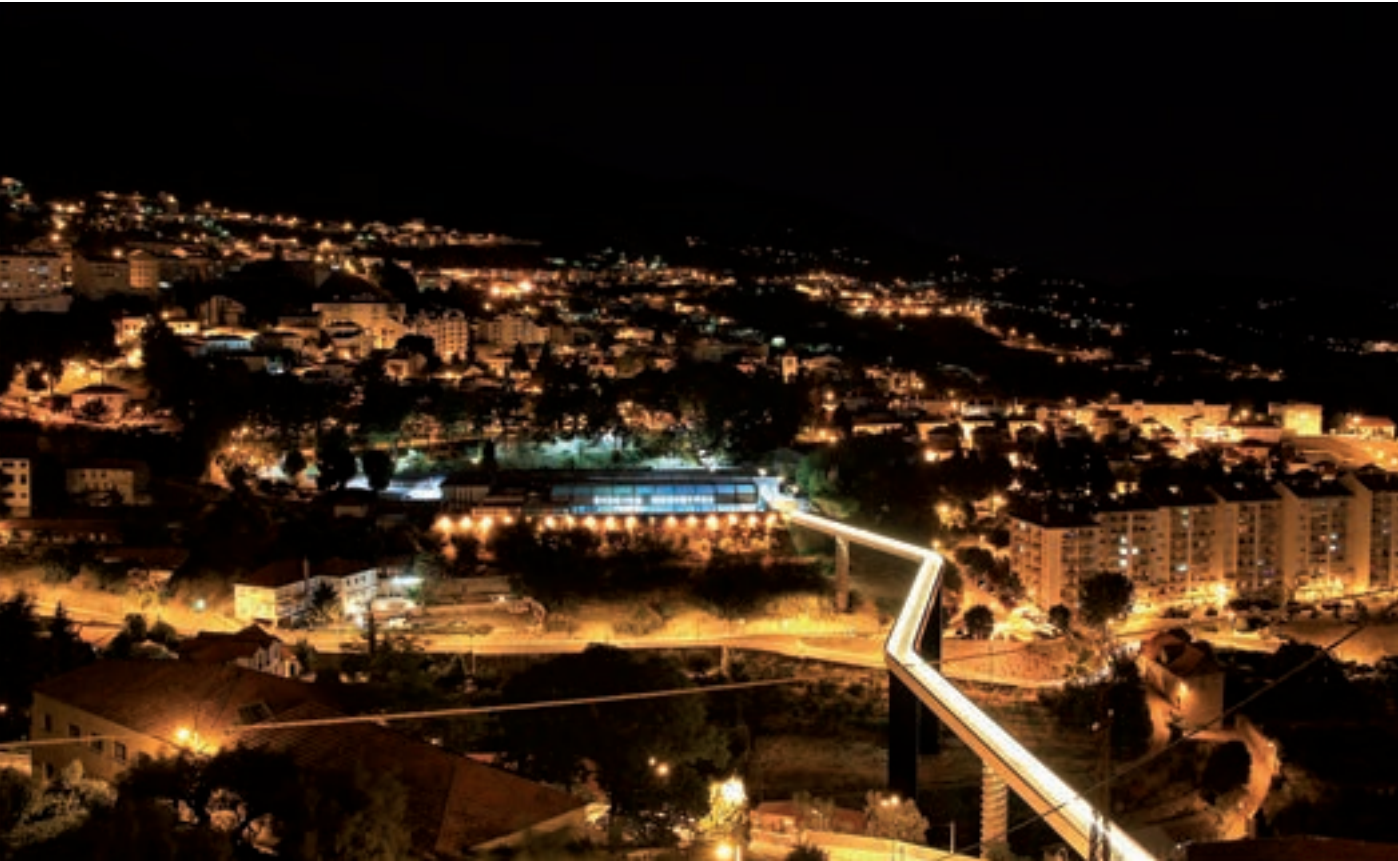
Bridge over the Carpinteira stream, Covilha, Portugal
