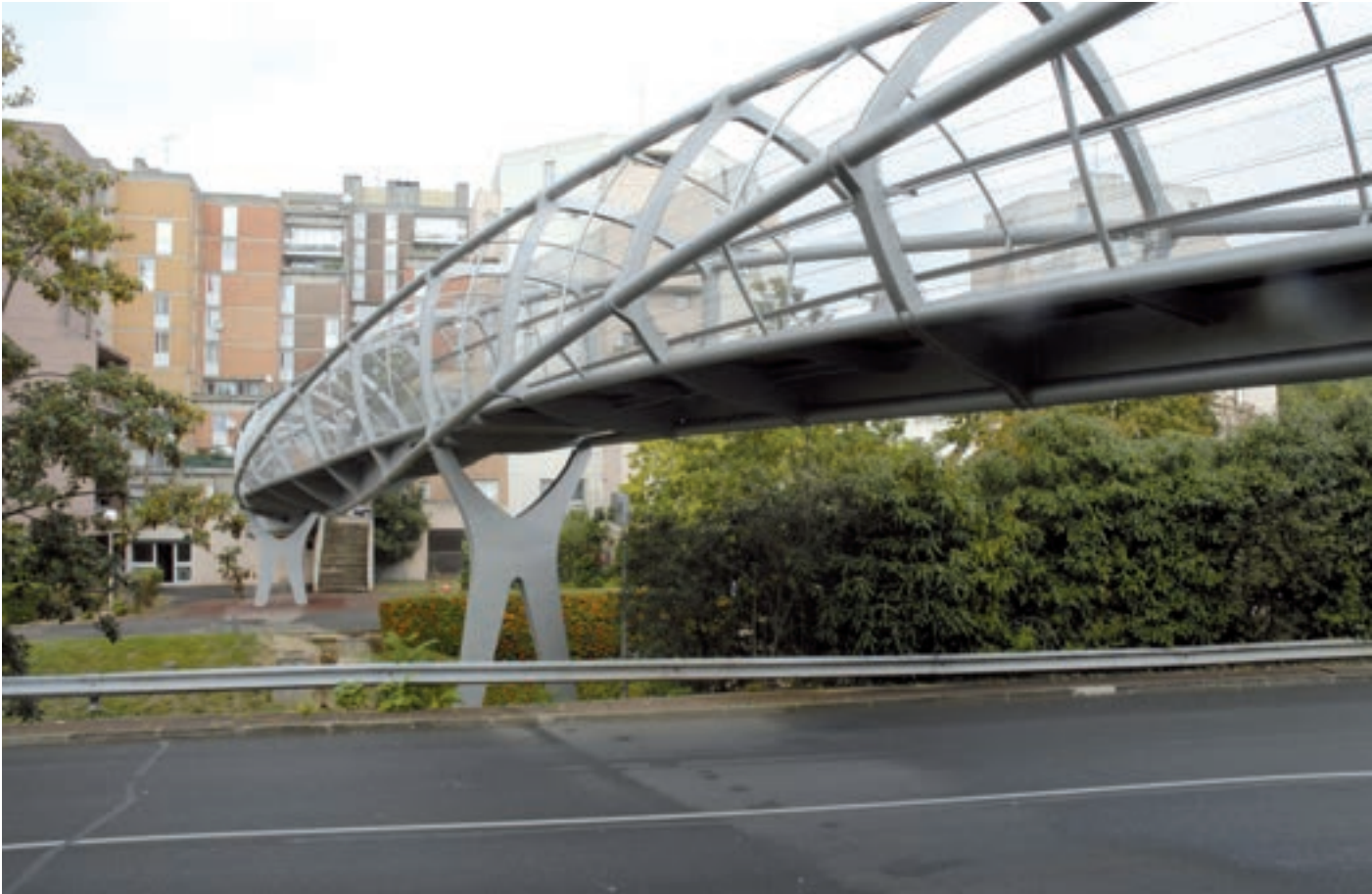
Footbridge over the inner ring road in Paris at Évry (arch. DVVD)
