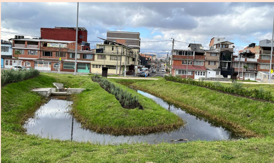
Pic. 3: AMB Project ‘Comprehensive Water Management for Adaptation to Climate Change in Metropolises Bogotá, Colombia
